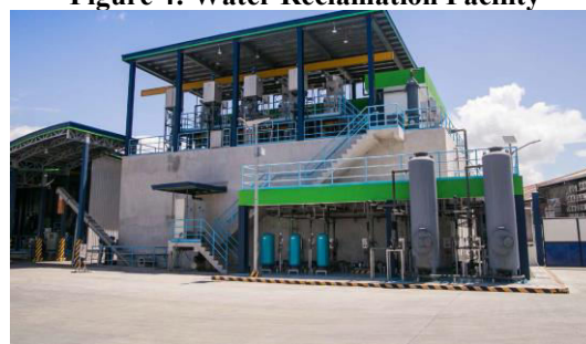
Figure 4: Water Reclamation Facility
