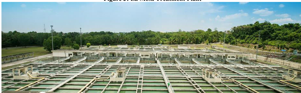
Figure 3: La Mesa Treatment Plant
